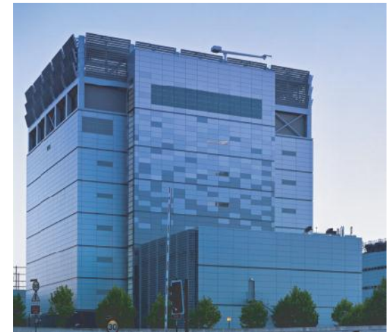
Rechenzentrum Telehouse Docklands
